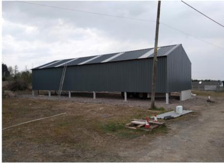
April has seen a lot of progress as many of you will have seen on Face Book. The whole structure is now complete with sides, roof and windows. Next to come are the concrete floor and land drains followed by the two roller doors.
