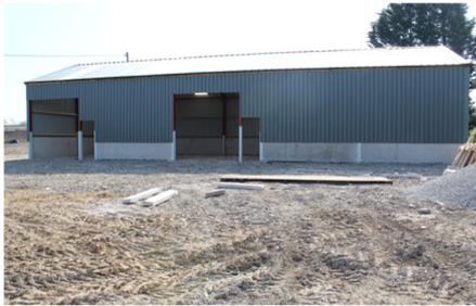
This is the front view showing where the doors are to be fitted. There is quite a large area in front of the building which will be levelled and covered in tar planings. There will also be a security fence on the right hand side.
